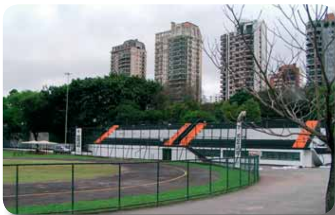
There are several rooms inside the big concrete spectator stand at the circles in Ibirapuera in Sao Paolo.
